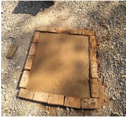
Fig. 6. Levelling of ground
