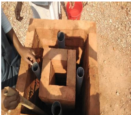
Fig. 8. Pipe installation and cavity filling
