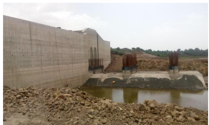
Weir body wall & piers of Anteshwar barrage Photo 2
