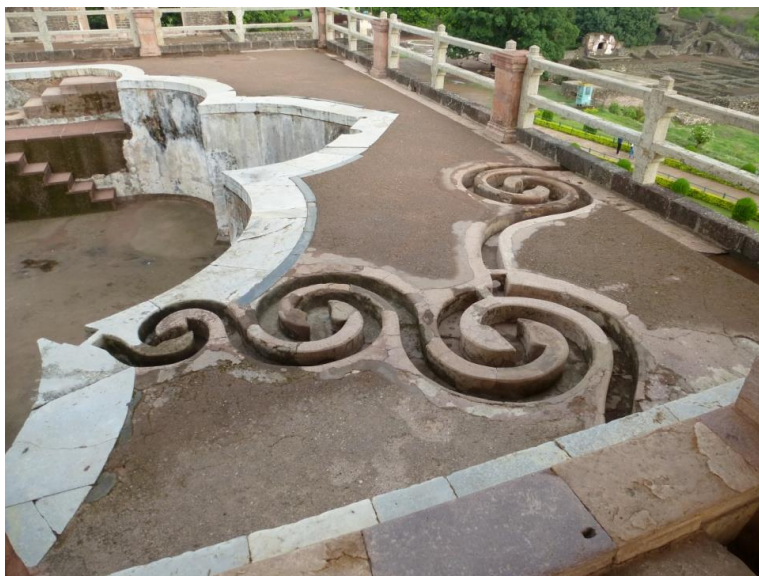
Intricate water channels to help sedimentation of suspended particles in water while slowly distributing the water, Mandu Fort, Jahaj Mahal, Madhya Pradesh
