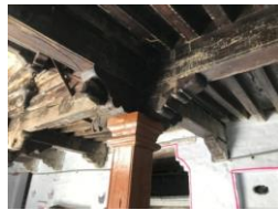
Fig7. Column and Beam Junction
