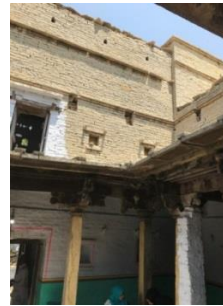
Fig16. View Of First Floor
