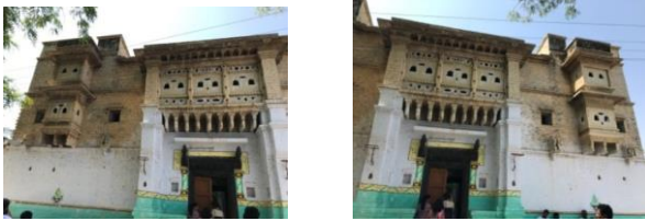
Fig11. Entrance Façade of the House
