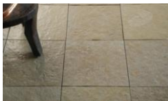
Fig5. Shahabad stone flooring
