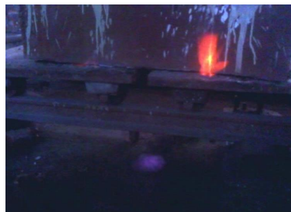
Fig. 9 Improper mould closing
