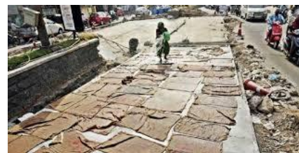
Fig.10- VDCC road construction at Hyderabad; source weblink- data:image/jpeg;base64,9j/
