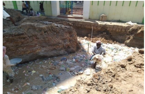
Fig-3: Plastic wastes are Spreading in the foundation
