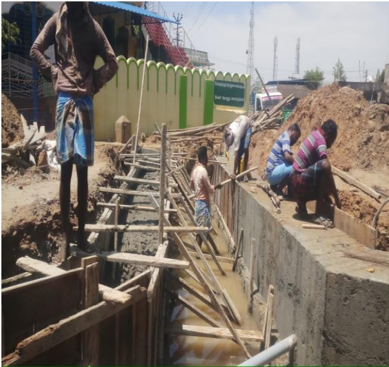
Fig-6: Culvert Body wall
