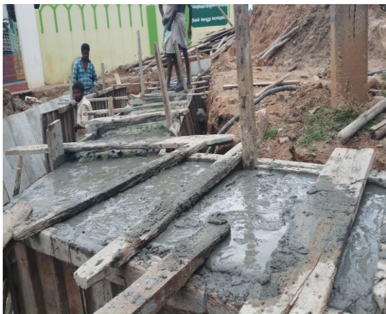
Fig-7: Side wall Concreting
