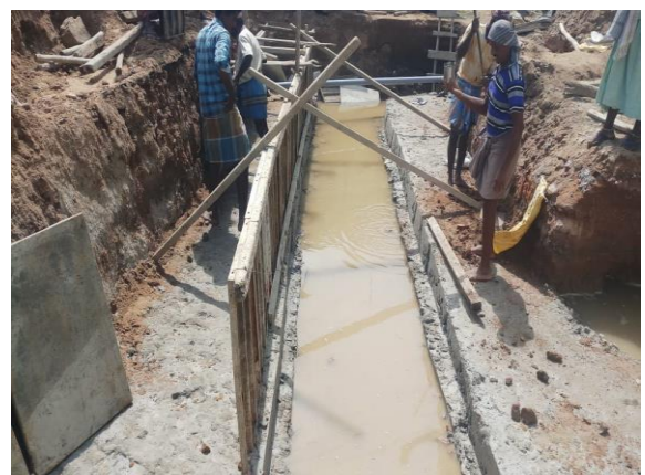
Fig-5: Body wall Centering progress
