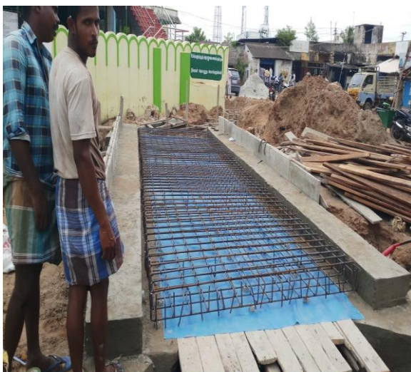
Fig-8: Deck slab Steel Fabrication
