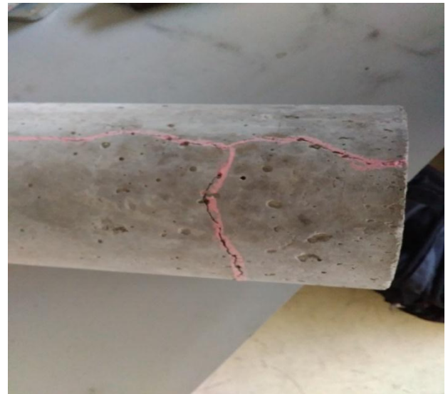
Fig. 4 Crack pattern of cylinder specimen after split tensile test
