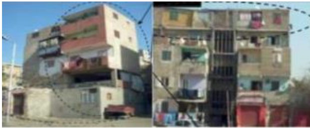
Fig-4- Vertical Intensification by increasing the number of Floors on the existing building to meet the needs of the population , source: Population- Based Solutions to solve the Housing Problem Through Expansion , D. Kamal Mahmoud Kamal Jiblawi
