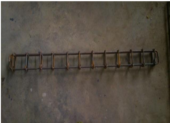
Fig.4. Reinforcement cage for flexural behaviour
