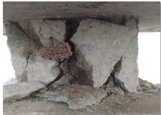
Figure 2: Failure of Concrete Sample
