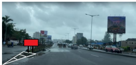
Fig.5. Information sign absent & Gore area marking absent.
