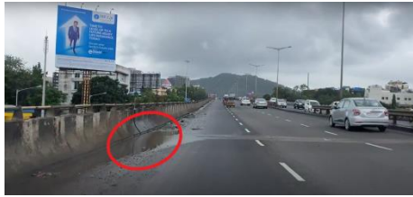
Fig.8. Clogged drains cause water-logging on road.
