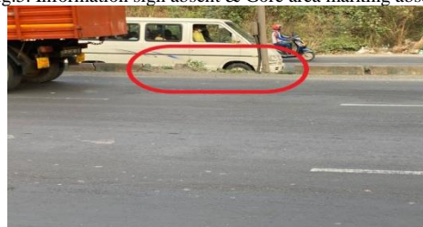
Fig.6. Broken median and misplaced barricade.
