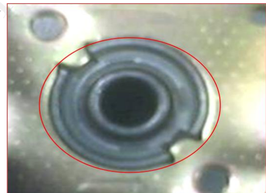
Figure 13 Gap observed between frame & Lower bearing assembly
