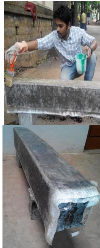
Fig 3 Applying Resin and GFRP
