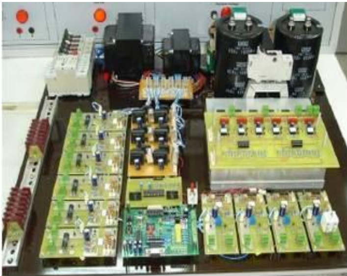
Fig. 8. Hardware setup for active power filter.
