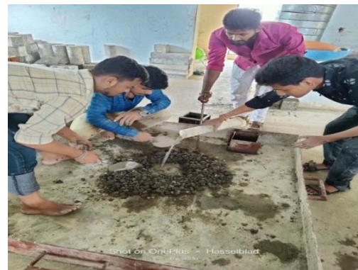
Fig 5. Mixing of Concrete
