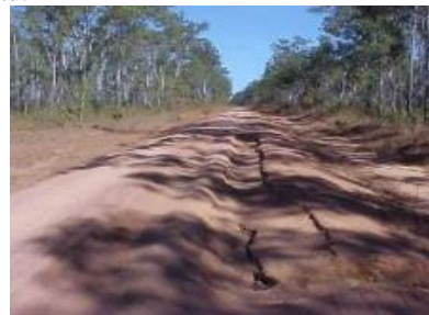
Rutting: A longitudinal deformation of a pavement surface formed by the wheels of vehicles. May be on a sealed or unsealed road.
