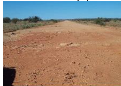
Rutting: A longitudinal deformation of a pavement surface formed by the wheels of vehicles. May be on a sealed or unsealed road.
