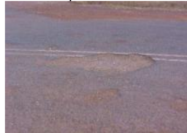
Pot Holes: Bowl-shaped depressions in the road surface, resulting from the loss of pavement material.
