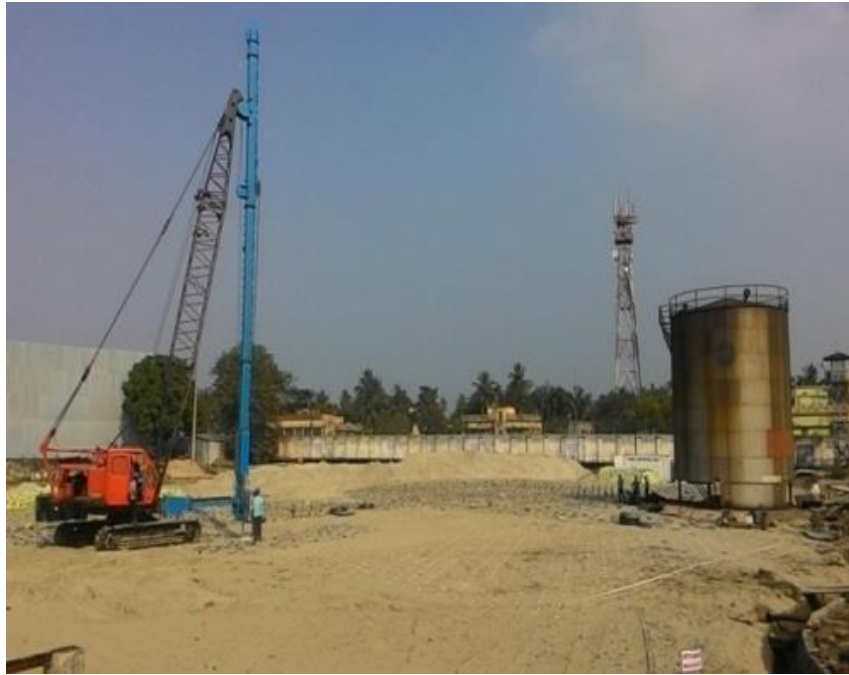
Fig.2. PVD installation is in progress at site.
