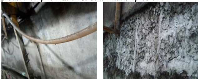
Fig-11: Concrete surface with (Left) or without (Left) using of 0.47 mm thick galvanized cold rolled color coated sheet in inner surface of shell concrete.
