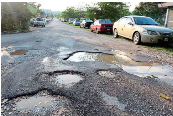
Fig. 3. Representative urban road surface with multiple potholes [35].
