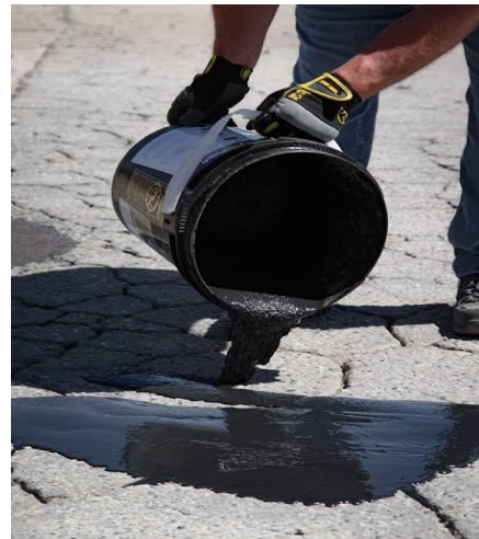
Fig.2: Alligator crack repair
