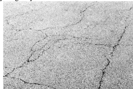
Fig.3: Block cracking
