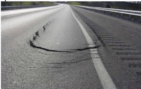
Fig.11: Slippage cracks
