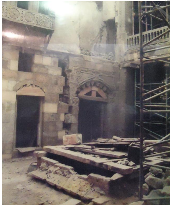
Figure 2. The Sinnary House before restoration
