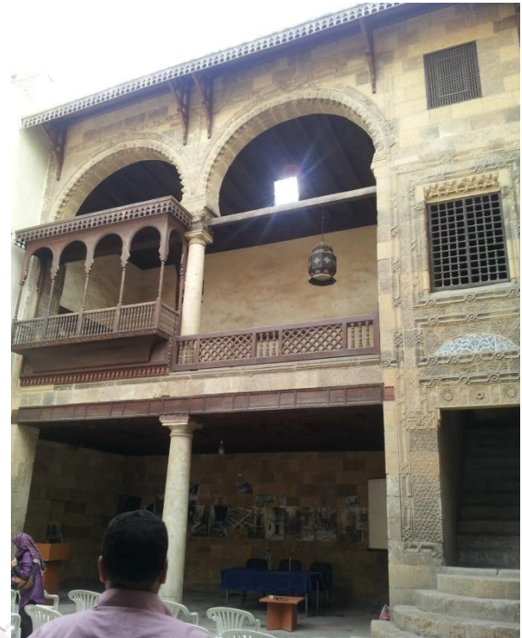
Figure 3. The Sinnary House after restoration
