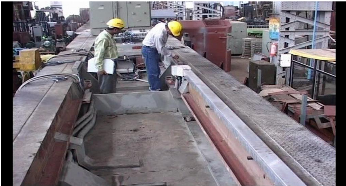
INSPECTION OF UNDERFRAME
