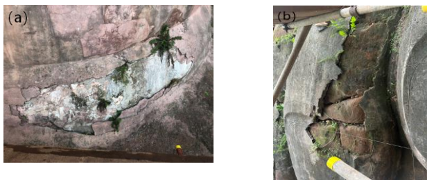
Fig 2 Deterioration status of Chuihui materials a. breast and abdominal reconstruction material failure, b. failure of hand repair materials
