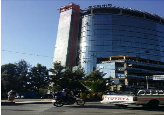
Figure 5. Camera set-up location for post office intersection
