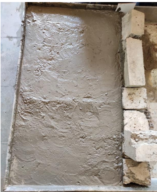
Fig.4 Laying of second layer of concrete
