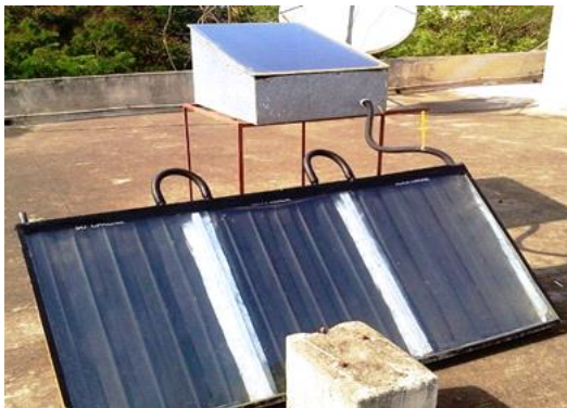
Fig 1: Free convection arrangement
