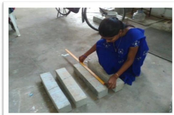
fig 3 measuring of crack distance
