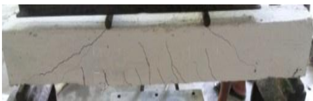
Fig.8 Typical crack pattern of shear beam specimen
