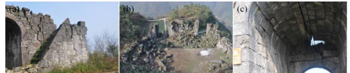
Fig. 1 Typical structural deterioration of Feifeng Castle a. Cracks and bulging on the south wall, b. Collapse of the north wall, c. Loosening of the arch
