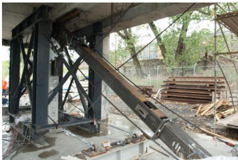
Fig. 13 - Building retrofitted using steel frames
