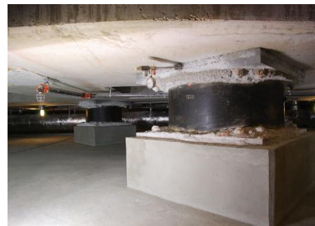
Fig. 15 - Lead Rubber Bearings
