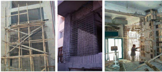
Fig. 12 - Cast-in-place infill walls
