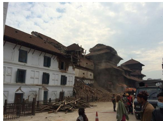
Fig. 1 - Damage at Durbar Square, Kathmandu after Gorkha earthquake
