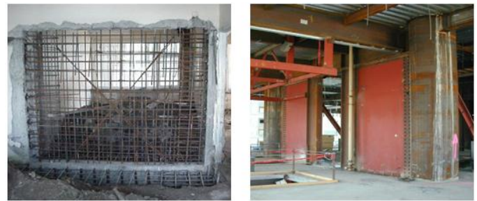
Fig. 11 - Adding Shear Walls to existing structures
