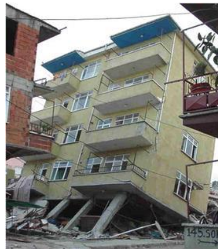
Fig. 3 - Soft story collapse in 1999 Kocaeli - Golcuk earthquake [2]
