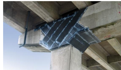
Fig. 8 - Polymer composite application
