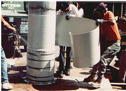
Fig. 10 - Installing Prefabricated Fiberglass jacket [11]
