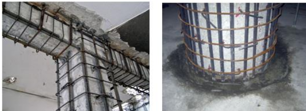
Fig. 6 - Column retrofitting by concrete jacketing [3]
