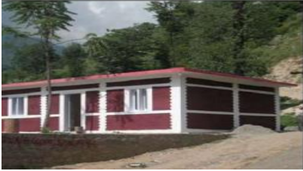
Fig. 8. Confined masonry structure defined seismic reinforcement
