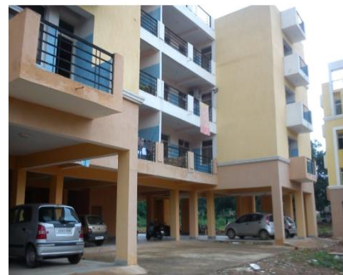
Fig 1. A typical OGS building located at Rourkela
