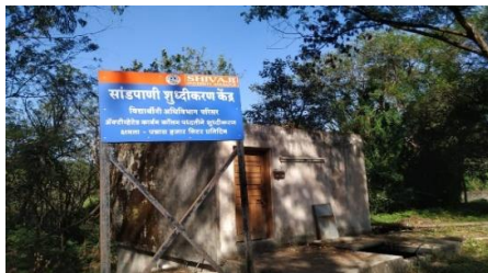
Fig. 8 Activated Carbon Column Method Treatment Plant in Shivaji University
