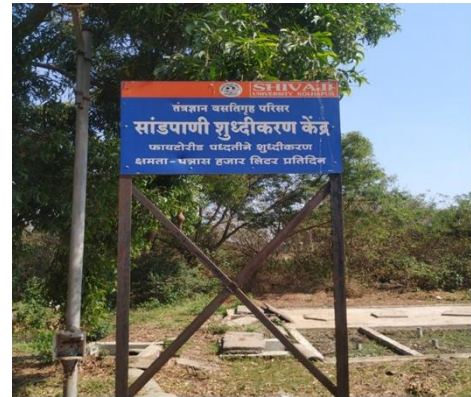
Fig. 4 Phytorid Treatment Plant
