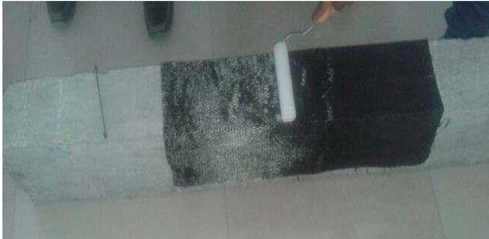
Fig. 3.5 Roller Used For Removal of Air Bubbles
