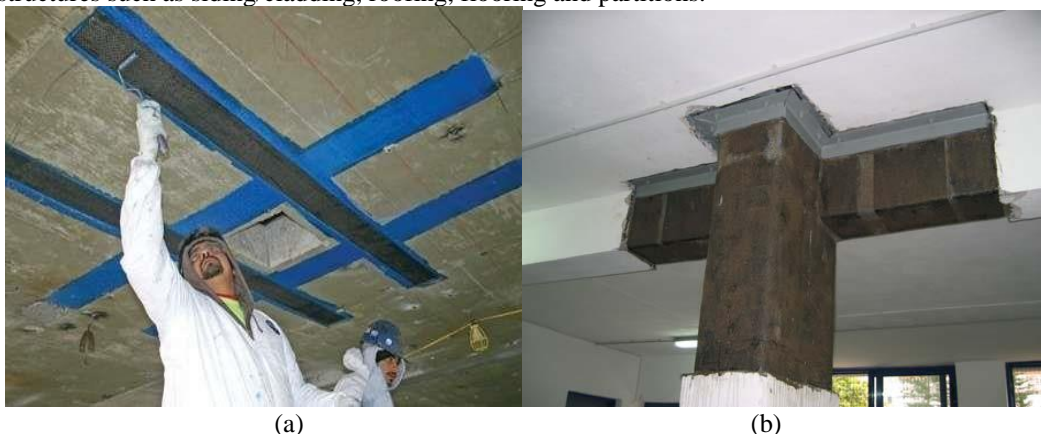
Figure.1.1 (A). Application of Externally Bonded FRP Composites. Figure 1.1 (B). Retrofitting Of Column-Beam Joint.
