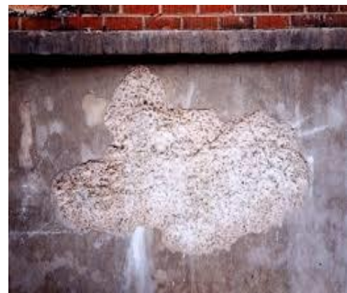
Picture 1 (Spalling of Concrete)
