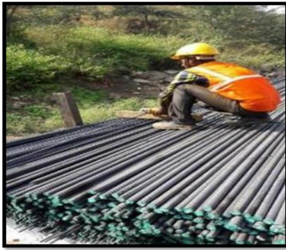
Stacking of Stirrups on Wooden Plank in Steel Yard.
