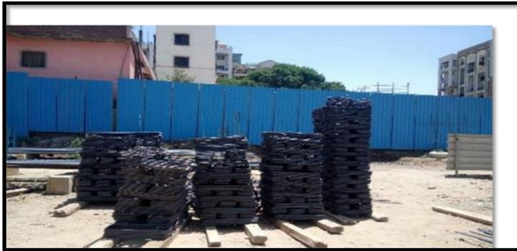
Stacking of Stirrups on Wooden Plank in Steel Yard.
