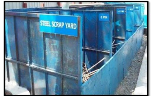
Diameter Wise Re- Steel Scrap Yard Bin
