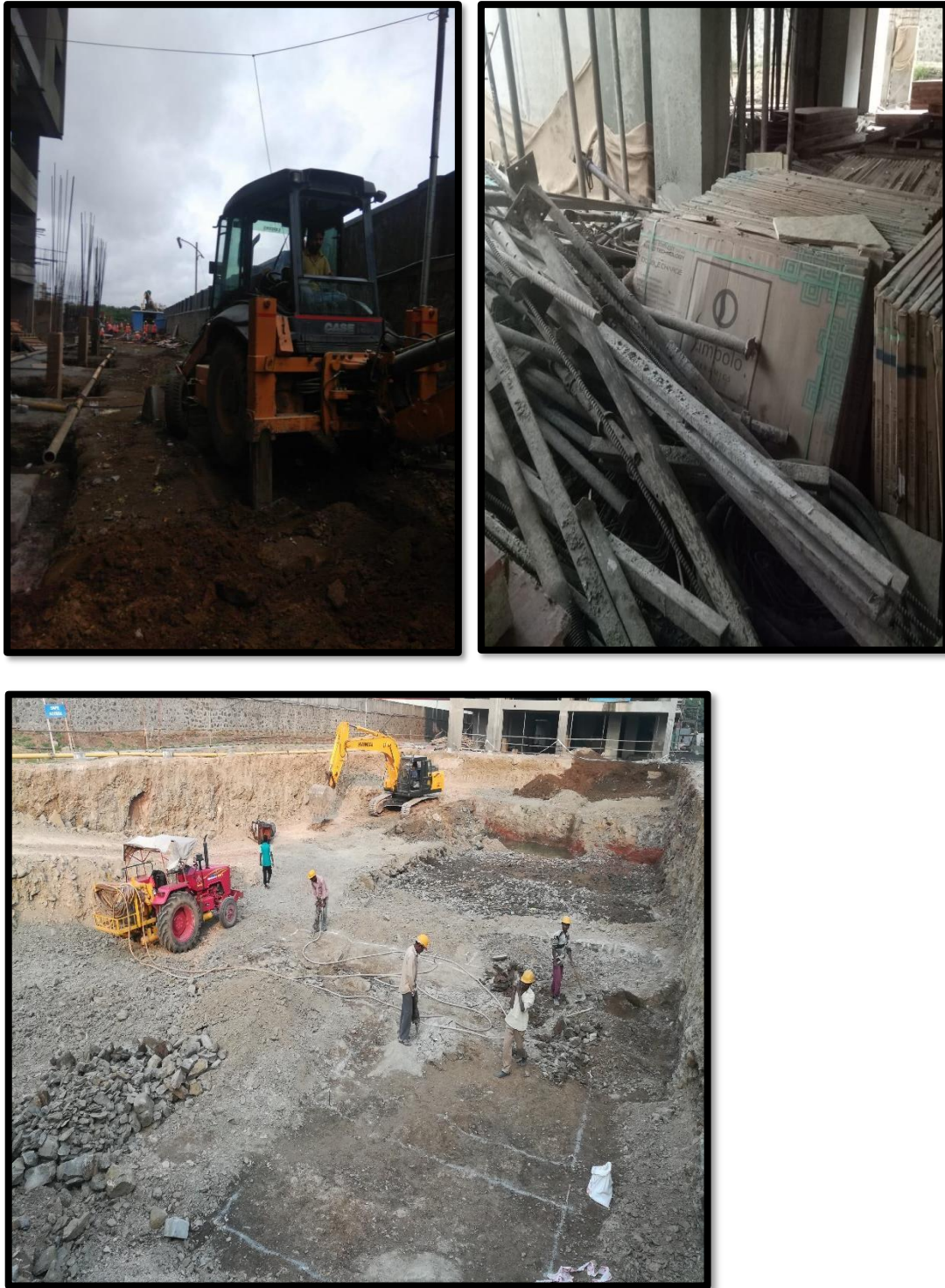
Fig 3.4 Site Observation Pictures – Project PQR
