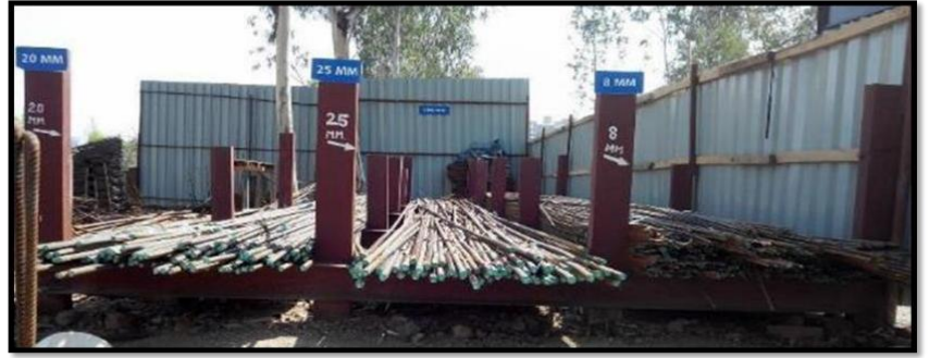
Steel Stacking In Racks For Each Dia. Of Bar
