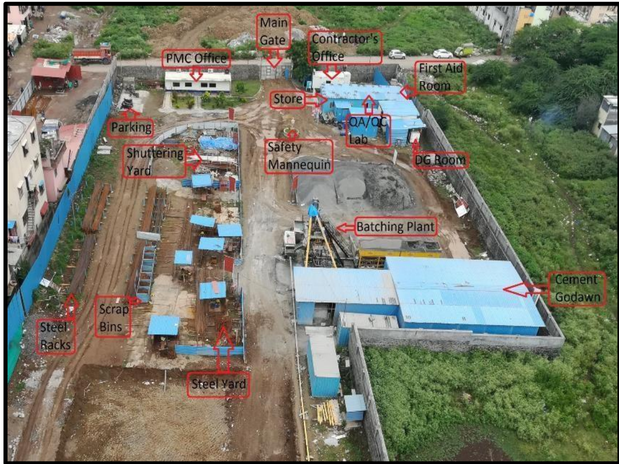
Fig 3.2: Actual Photograph of Logistics at Site ABC
