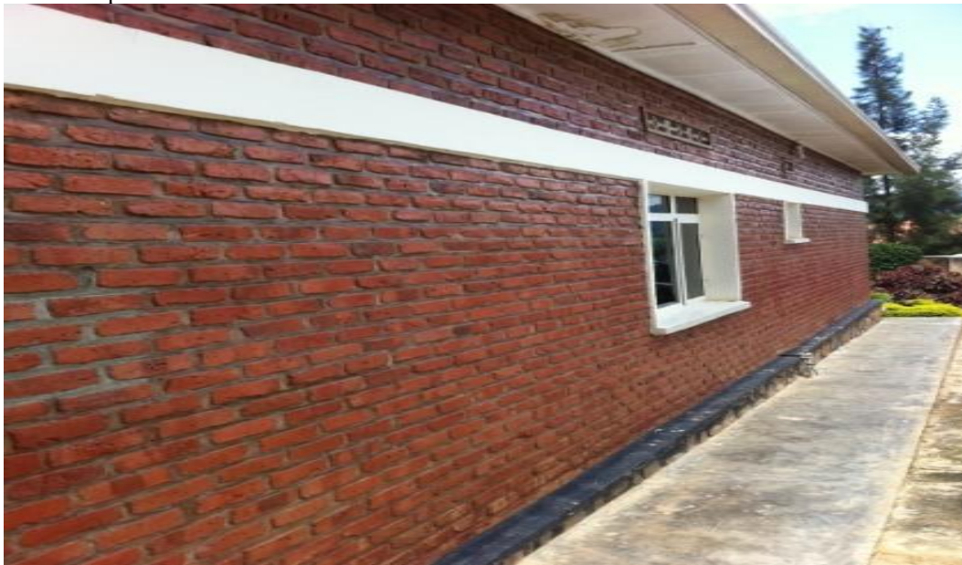
Figure 4. Typical formal house wall made of fired brick [55]
