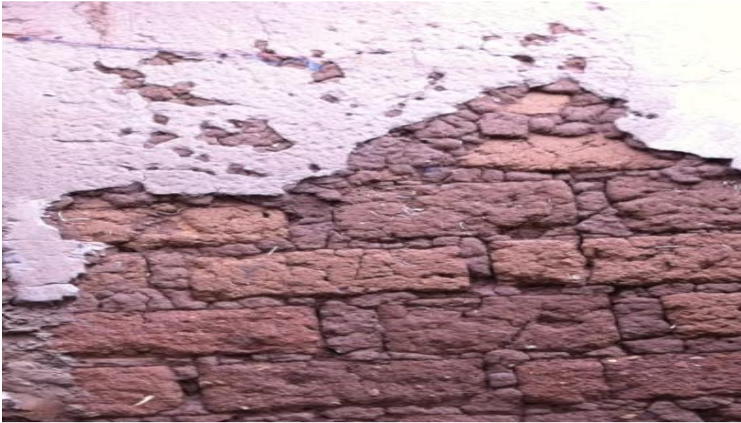
Figure 3. Typical informal house wall made of mud brick [55]
