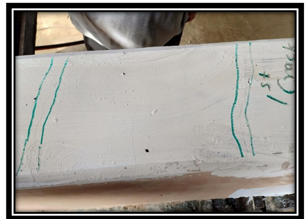
Figure1 : Crack Propagation at Center Top
