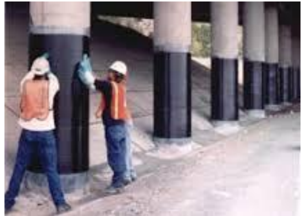
Fig.1 Wrapping of FRP.
