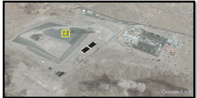
Fig.8: Oman Landfill Location
