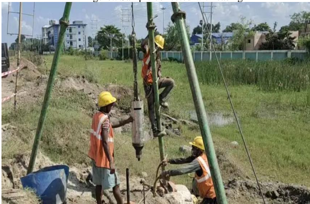
Figure : SPT being conducted at Site.
