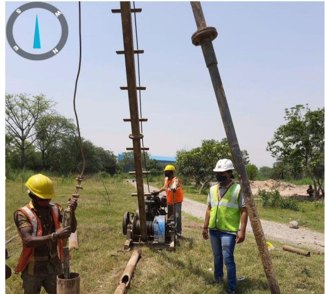
Figure: SPT being conducted at Site.
