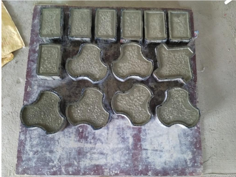
Figure-2- preparation of paver blocks
