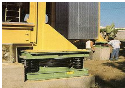
Fig. 1.Spring Base Isolator Structure [8]
