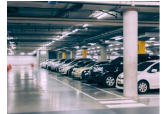
Fig 1.2 Underground parking structure
