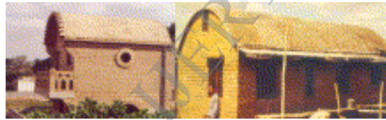
Figure 20: Vaulted roof building made of stabilized mud blocks
