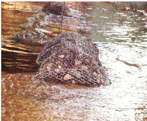
Fig 8. Sub aerial breakwater
