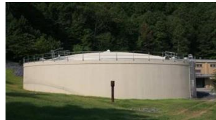
Fig.2. Equalization Tank
