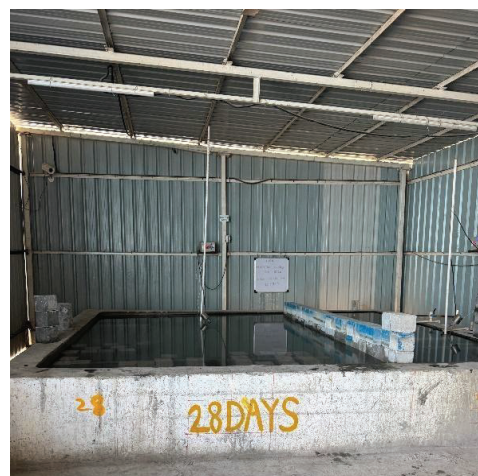
Figure 7: Casting of the concrete and curing
