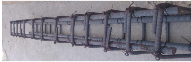
Figure 7 Reinforcement cage
